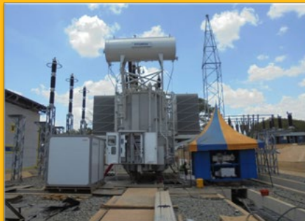
9000l/hr Oil Filtration Machine with 2140 m3/hr Double Stage Vacuum Pump
