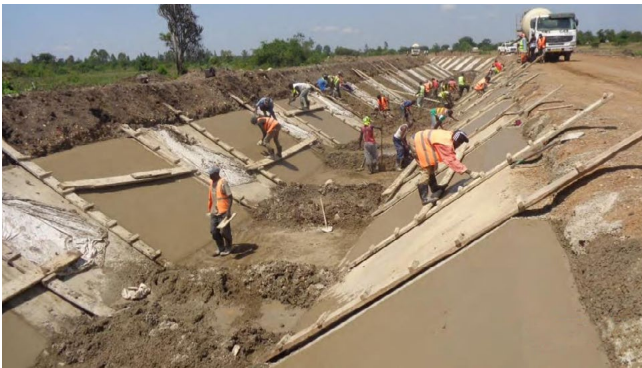
On-going construction of the main canal for conveyance of water from the water intake point. (Photo Courtesy - NIA)
