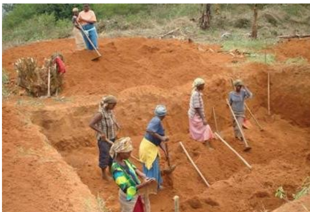
Digging of rectangular pits for rain water harvesting
