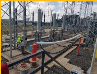
Testing using 330 kV Series Resonance Tester, 30 - 300 Hz at Thika Road 220/66 kV GIS Substation
