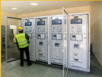
Testing and Commissioning of Efacec Protection Panels at 132/33 kV Naivasha Substation
