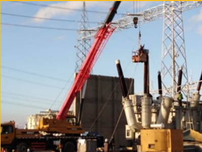
Installation of 200 MVA 400/220/11 kV AutoTransformer at Isinya 400/220 kV Substation
