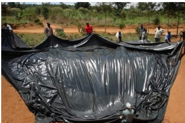
Lining of the pits with a butyl rubber membrane to prevent seepage of harvested rain water.
