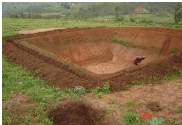
Digging of rectangular pits for rain water harvesting
