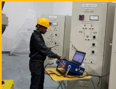
ARM Engineer commissioning at 132/33 kV GIS Substation in Basrah - Iraq
