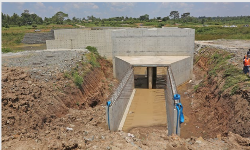
Intake section connecting intake to the headworks canal in Lower Nzoia Irrigation Development Project (Photo Courtesy - NIA)
