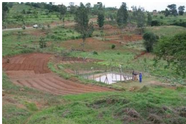
Lining of the pits with a butyl rubber membrane to prevent seepage of harvested rain water.
