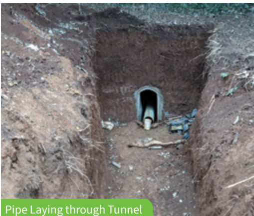
Installation of Precast Concrete Lining
