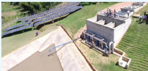
Figure: Solarized power configured with grid to power Kaimosi Water Treatment Plant
