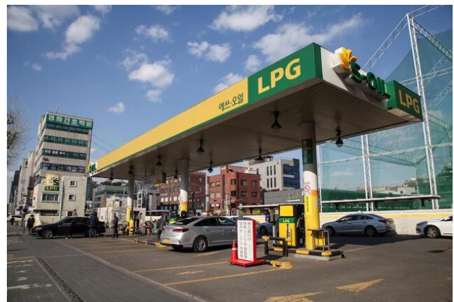
Figure 1; Seoul LPG taxi refueling station
