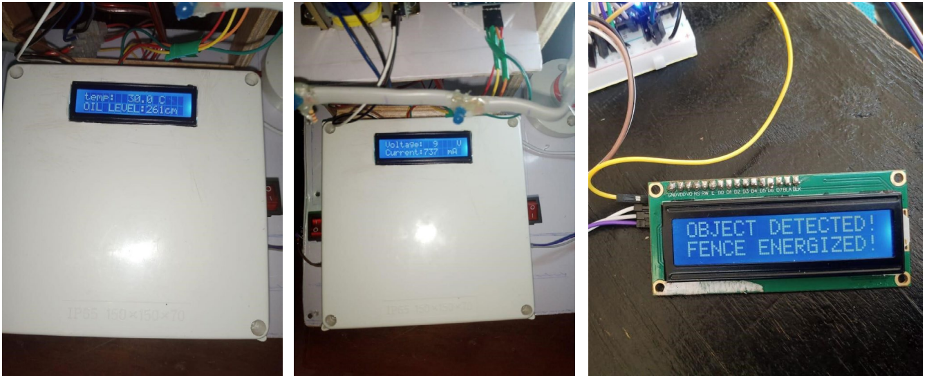
Figure 3: The anti-the Figure 5: Temperature, Oil level, Voltage and Current monitoring results ft subsystem system during construction stage
